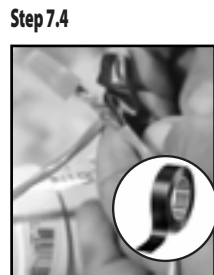
Secure the wire nuts with electrical tape.
